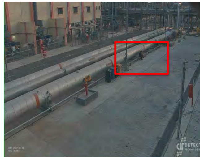
Observation: HC: Unsafe Act: Person found sitting on pipe
