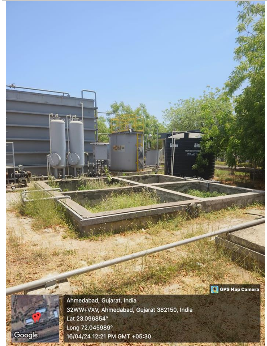
Figure 11: Geotagged Photographs of STP
