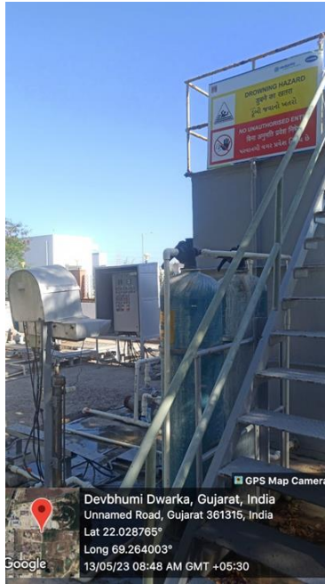
Figure 11: Geotagged Photographs of STP
