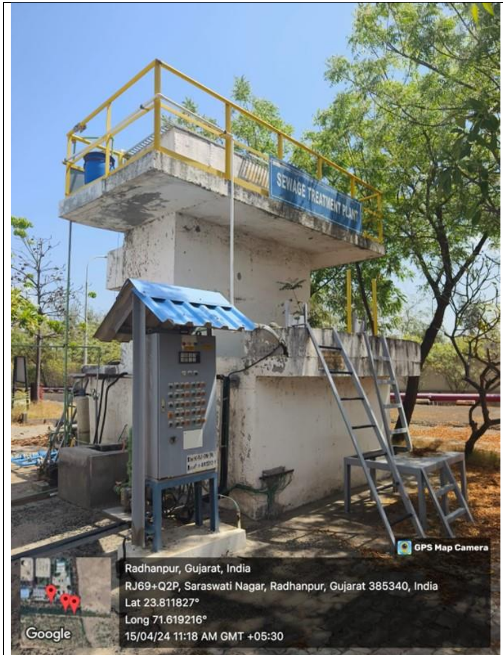
Figure 11: Geotagged Photographs of STP
