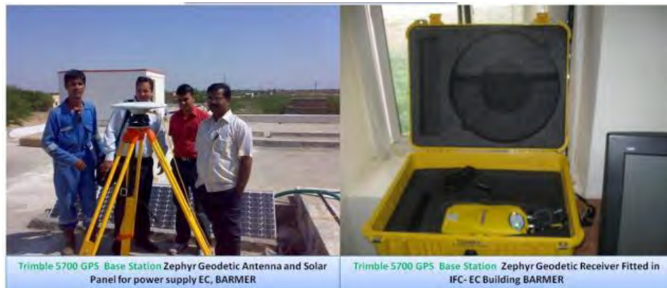
Figure 4: Base station is located on top of IFC EC centre and fitted with Trimble 5700 II receiver with Zephyr Geodetic antenna.
