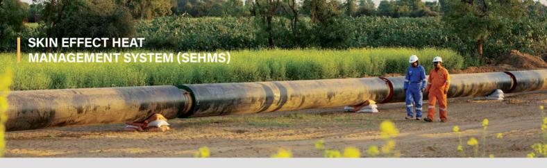
SEHMS technology is a proven electrical heating solution used for longdistance piping and pipelines.
